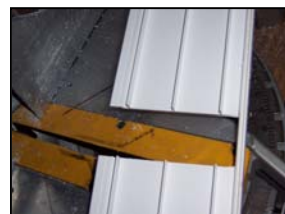
Cut a 3-7/8" notch for a 4" piece (or a 5-7/8" notch for a 6" piece)
