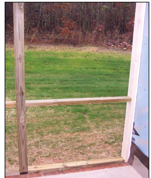
Cut a 3-7/8" notch for a 4" piece (or a 5-7/8" notch for a 6" piece)
